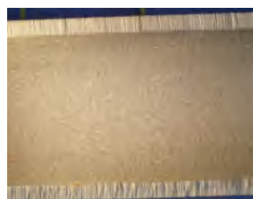
The wall after mechanical cleaning, no pitting or corrosion on the pipewall.
