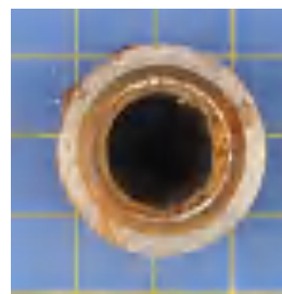
on the exterior with minor rusting, a small amount of deposit was evident.
